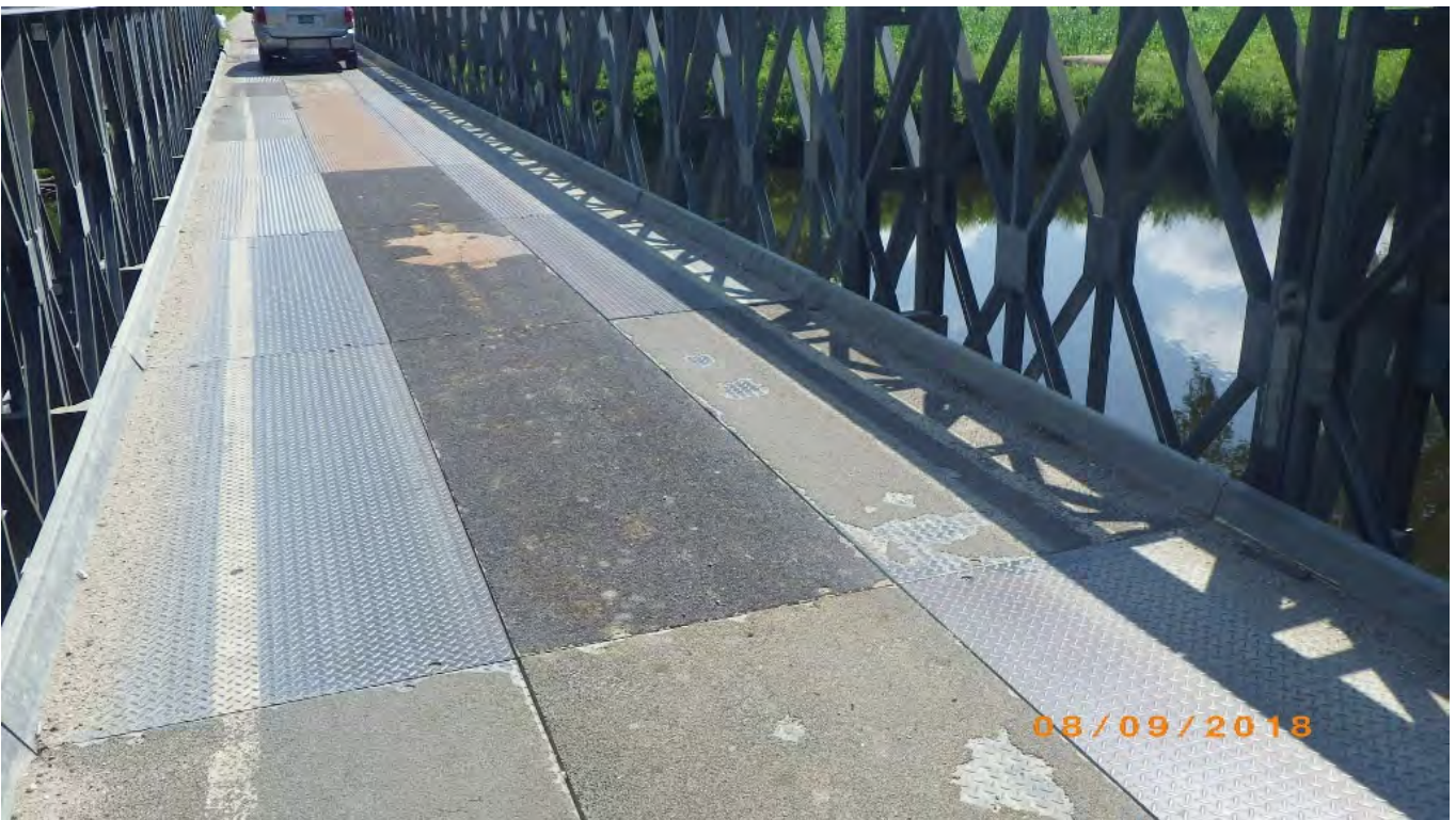
Picture four: Existing deck
