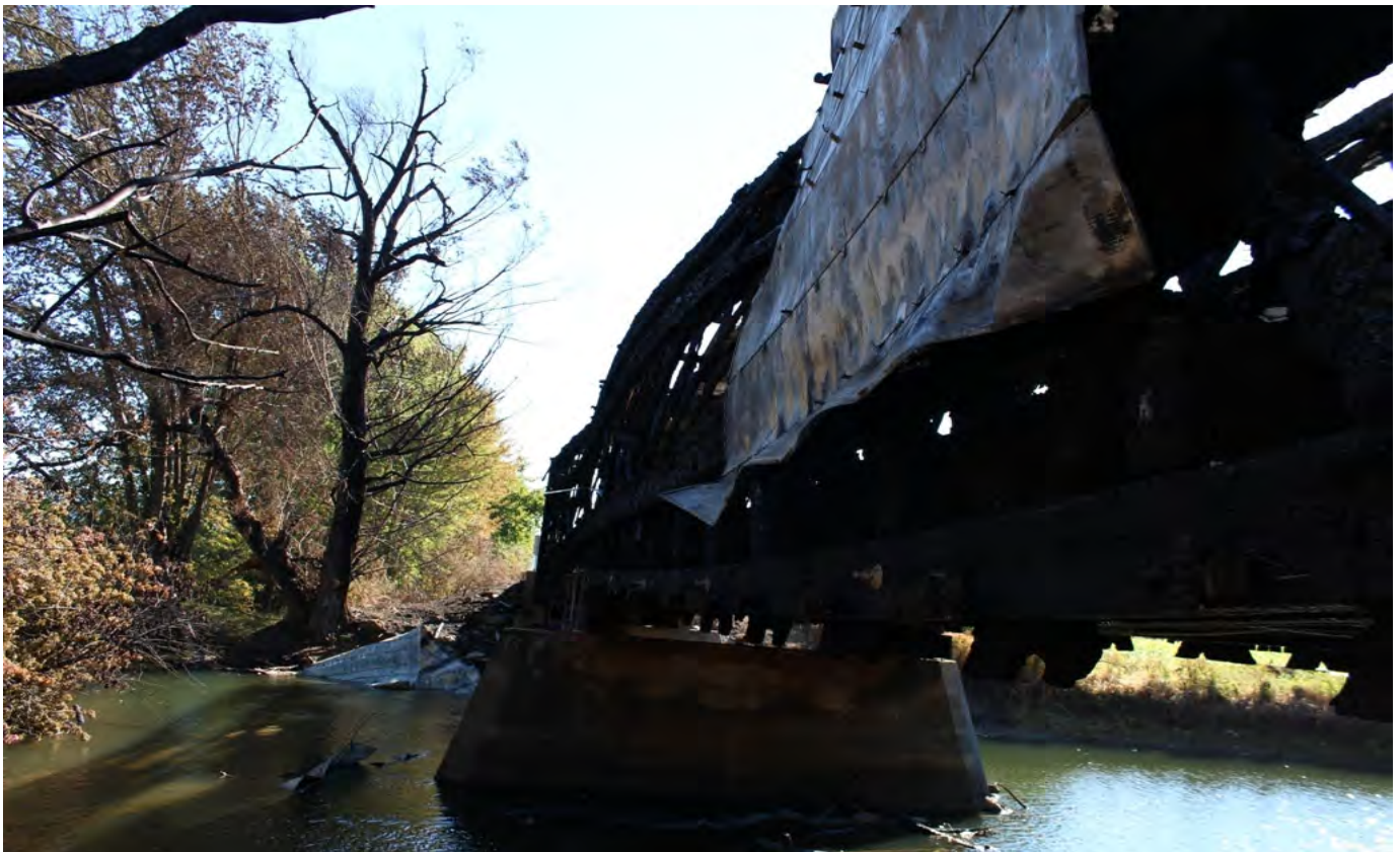
Picture six: Fire damage to existing center pier
