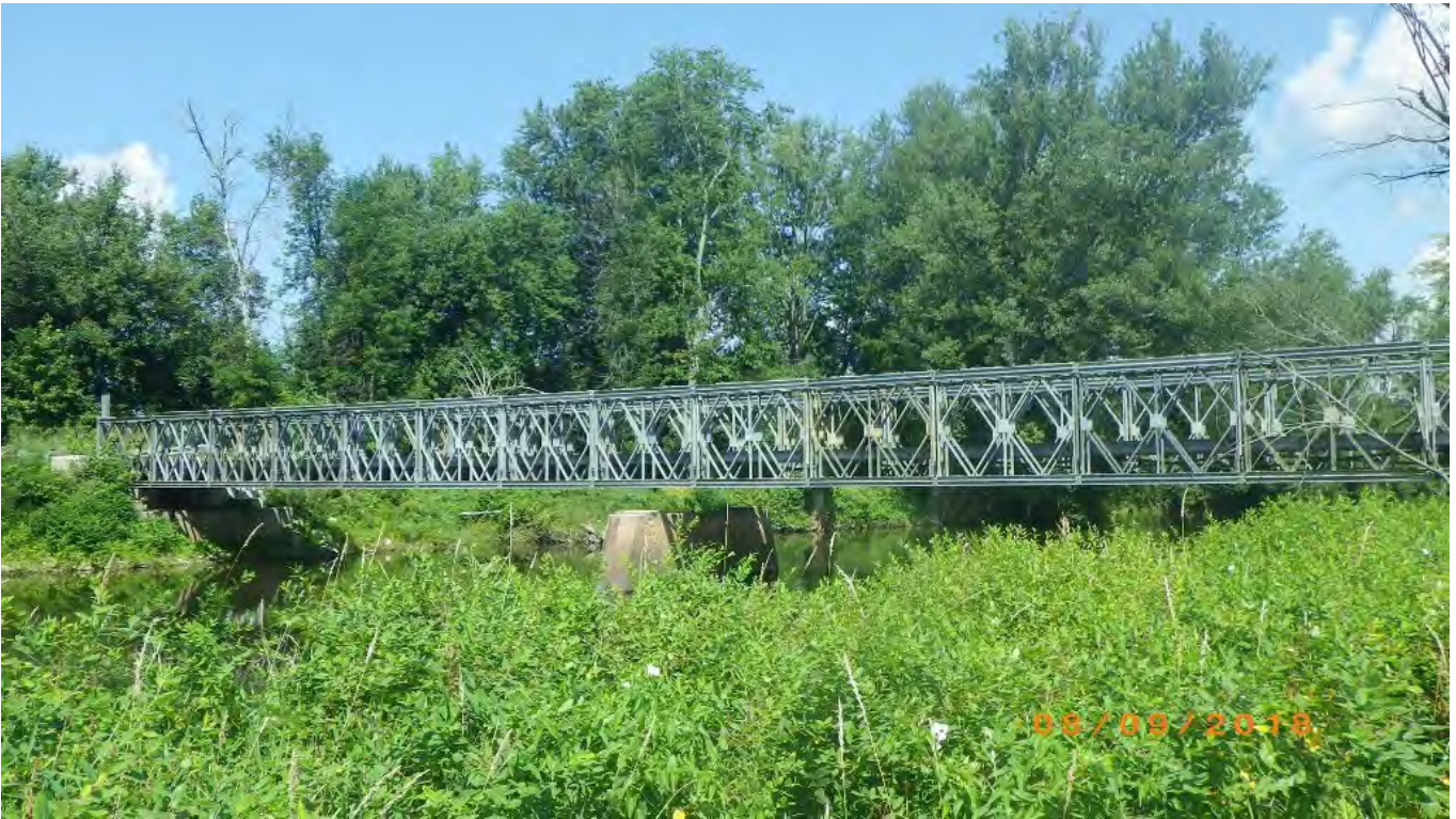
Picture three: Existing temporary bridge
