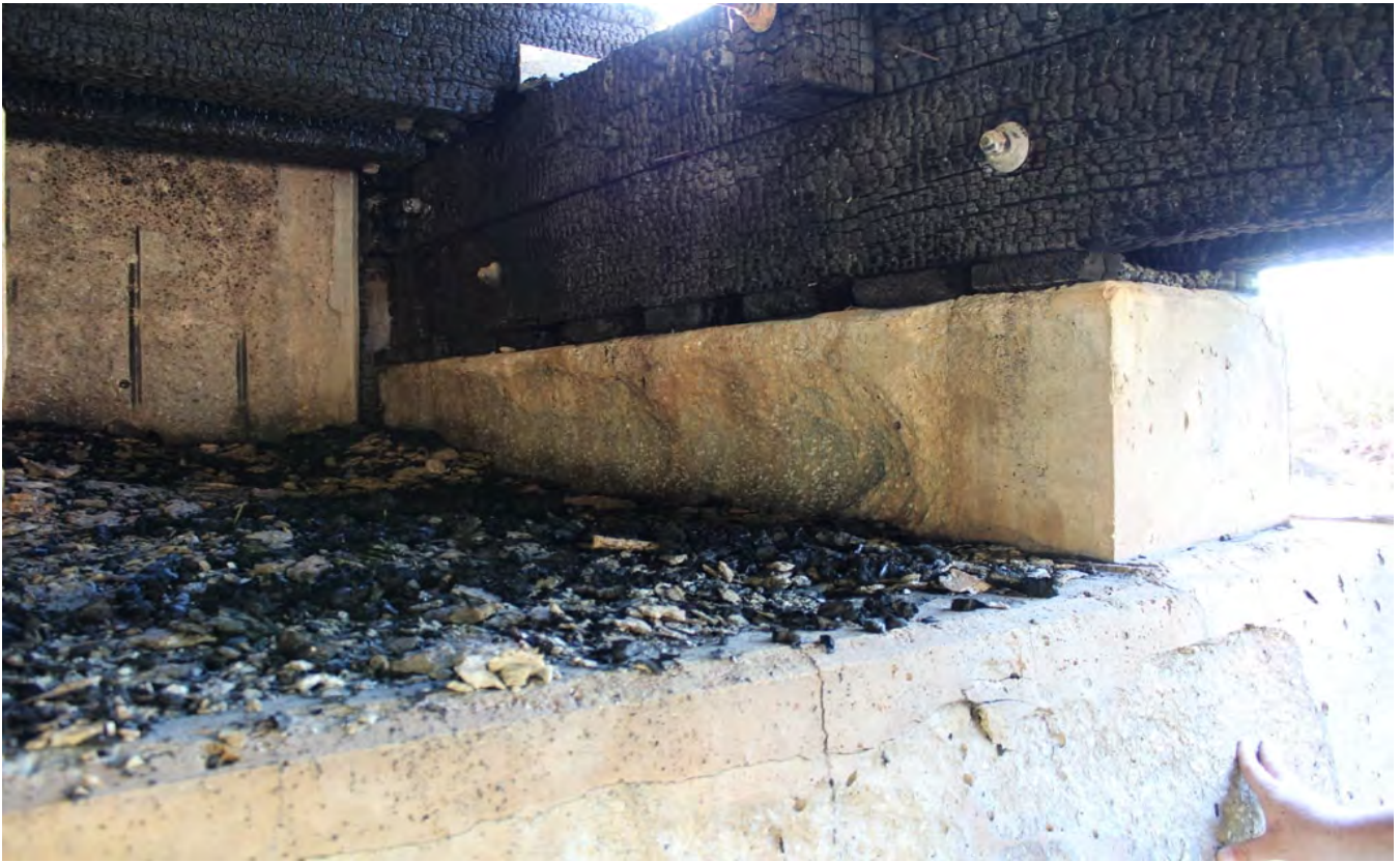
Picture five: Fire damage to existing abutments
