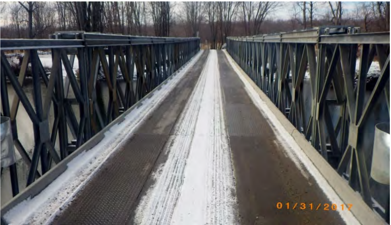
Picture two: Looking West over temporary bridge
