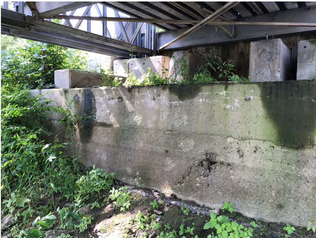
Figure 3.6: Facing western abutment.
