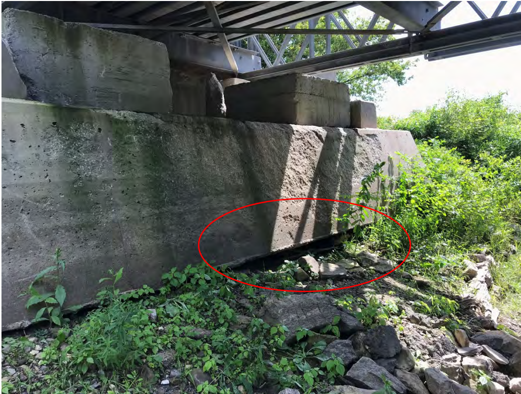
Figure 3.3: Facing eastern abutment; note material loss exposing bottom of abutment and spalling of concrete.
