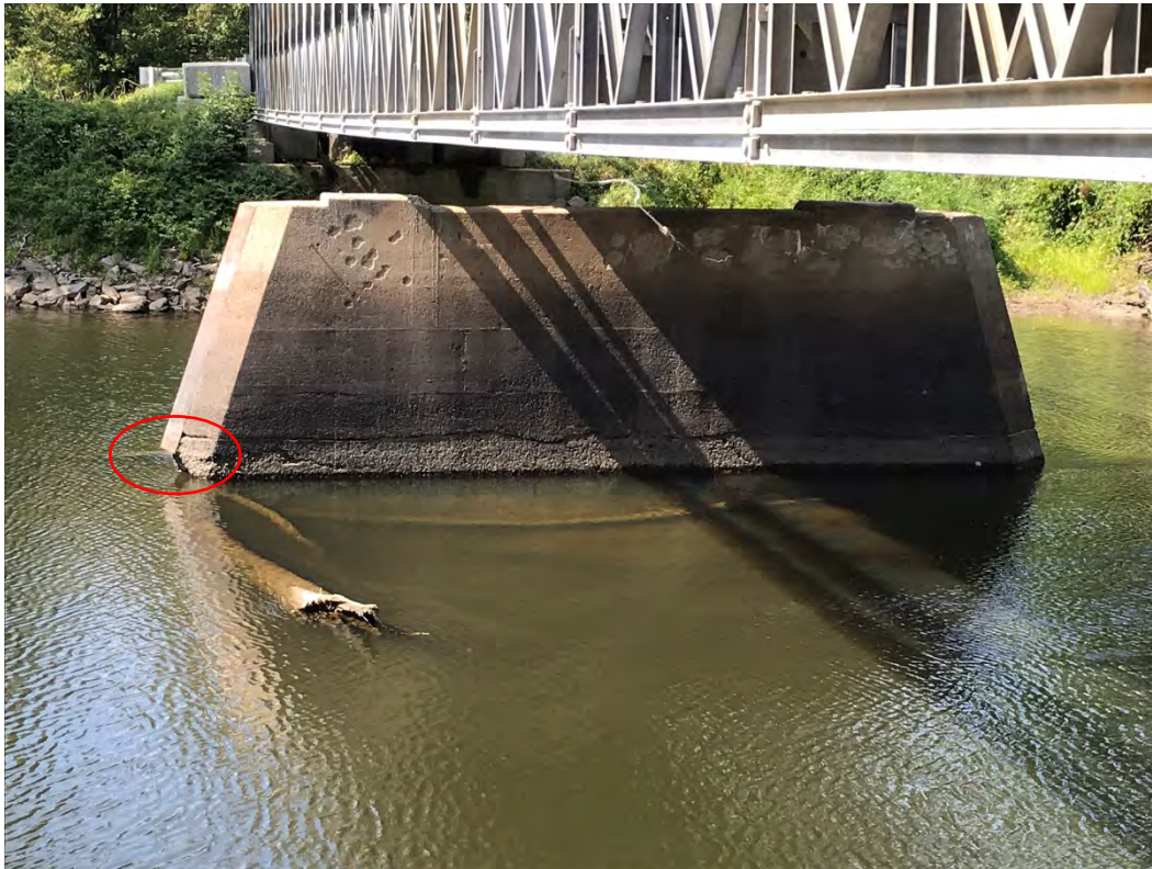
Figure 3.4: Facing west towards center pier; note spalling of concrete and exposure of bottom of pier. Temporary bridge is not connected to or bearing on pier.
