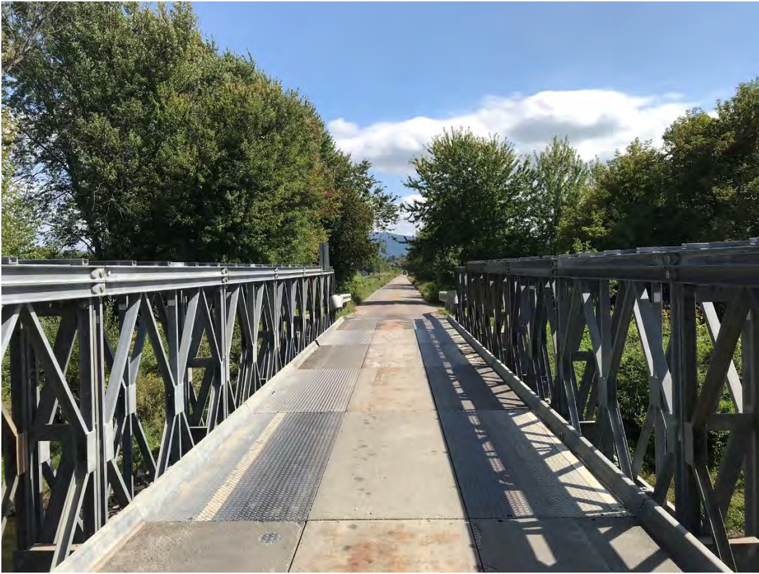
Figure 3.1: Facing east; note steel plate deck on temporary bridge.
