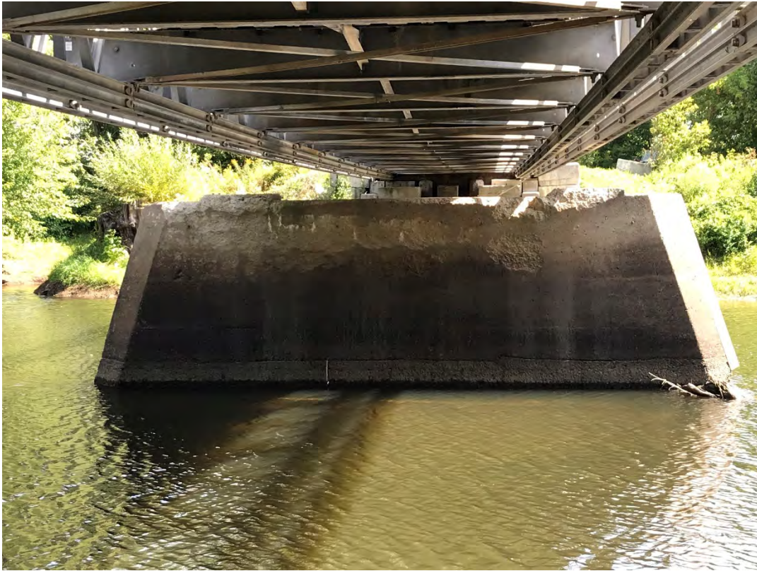
Figure 3.5: Facing east towards center pier; note spalling of concrete.
